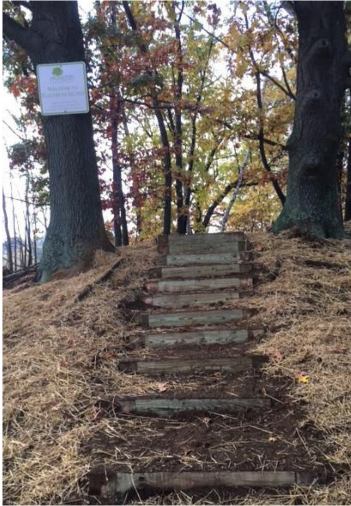
Box steps will control erosion and provide safer passage to Elizabeth Island trails.
